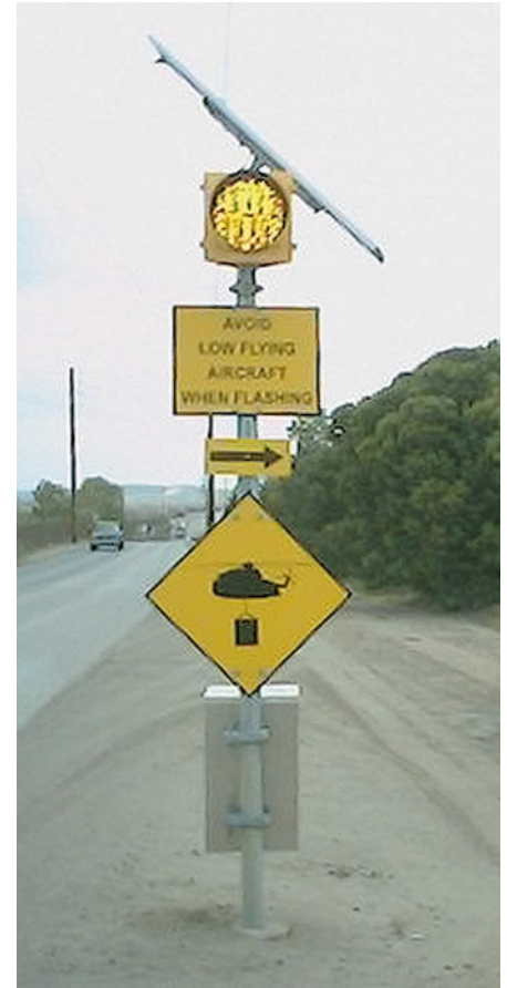
Flashing beacon warns motorists of low-flying helicopters.
