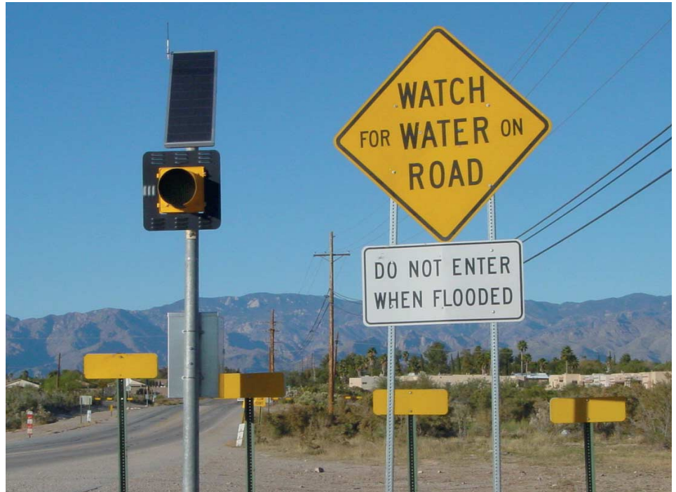
Solar-powered high-water flashers warn motorists of flooding at unbridged crossings.
