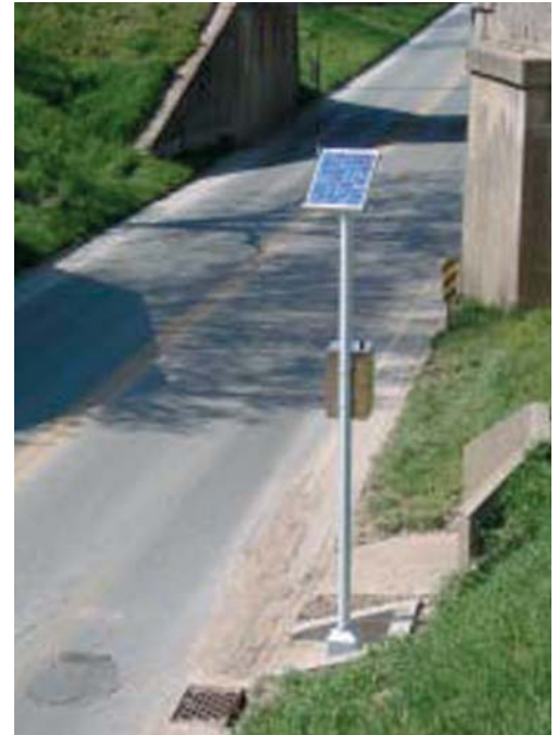
Sensor station assembly at the underpass
