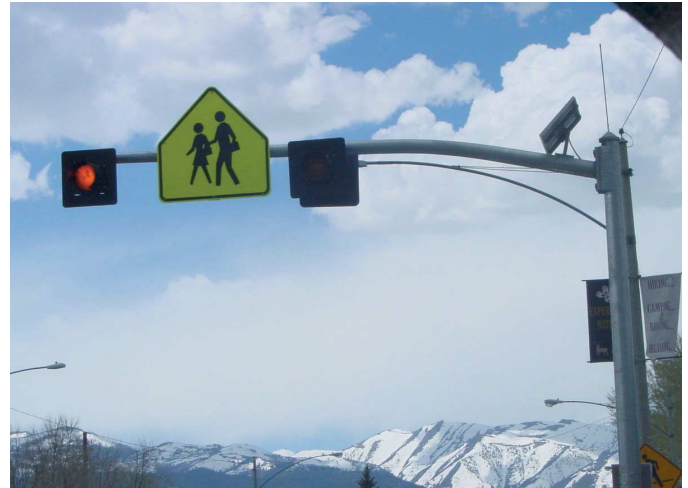
Dual application school/pedestrian-activated solar flashers
