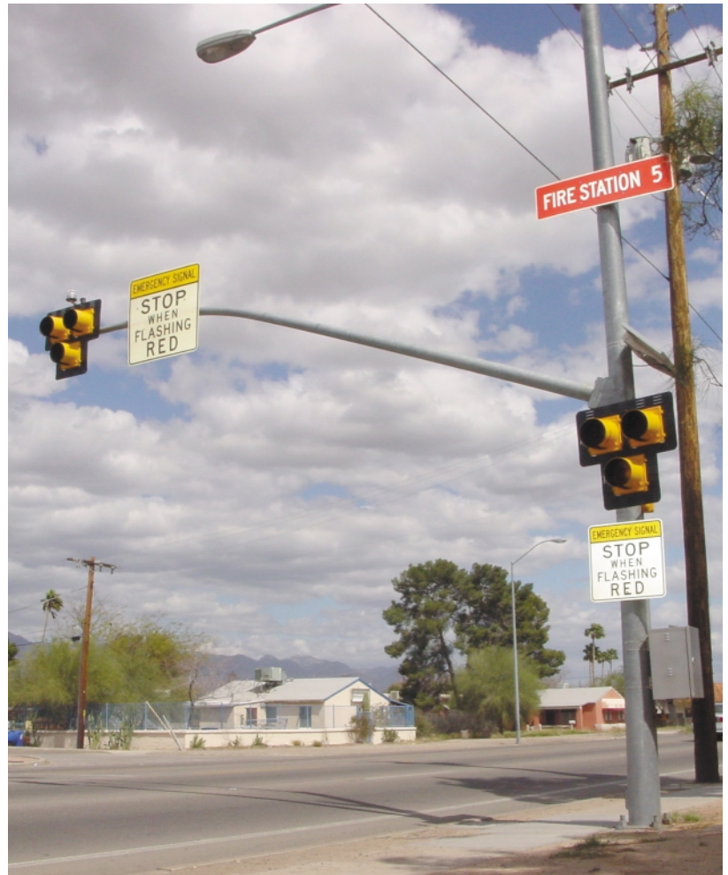
Tucson's Fire Station #5 with solar-powered flashing beacons.
