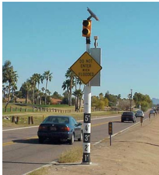
High-water warning system for flash flood area
