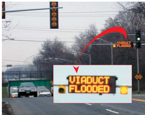
Matteson, Illinois "Viaduct Flooded" advance flashing beacon
