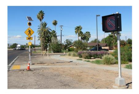
In lieu of adequate support from the manufacturer, STC stepped in to help improve the situation. Working with the town's traffic signal technician and Scouten Engineering, the town's contract traffic engineering firm, a solar Ped-X system was proposed at the crossing using STC 12-inch amber, DC LED lamps.
