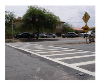
The project was configured by Parsons Brinckerhoff acting as a consultant to ADOT. The street has four through lanes of travel: a left turn and a 9-foot wide median. Acting as the southwest distributor for Traffic Safety Corporation, Solar Traffic Controls provided 12 - TS500 series fixtures for the project along with poles, flashing beacons, pedestrian button stations and a solar power package to run the entire system.
