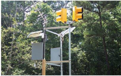
The system made use of STC's amber and red DC LED lamps which include high efficiency LED elements as the base light source. All the equipment had to be designed to accommodate special mounting
