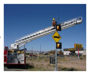
The flashing beacons were also outfitted with a clear confirmation beacon strobe so the fire truck driver could ascertain if the systems were active. Activation at this time is done using handheld transmitters installed in each of the vehicles. Future plans are to add a wall mount transmitter.
