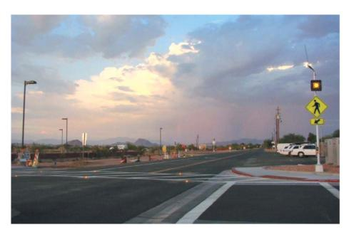
Working with a local engineering firm, STC personnel helped design and specify a suitable equipment package for the project. The package consists of a Traffic Safety Corporation 6-light IRWL with a solar power adapter. The solar power adapter is based on a design STC has manufactured for Traffic Safety for several years. It includes an LCD user interface screen with data collection and display, solid-state load control and a radio transmitter package.
