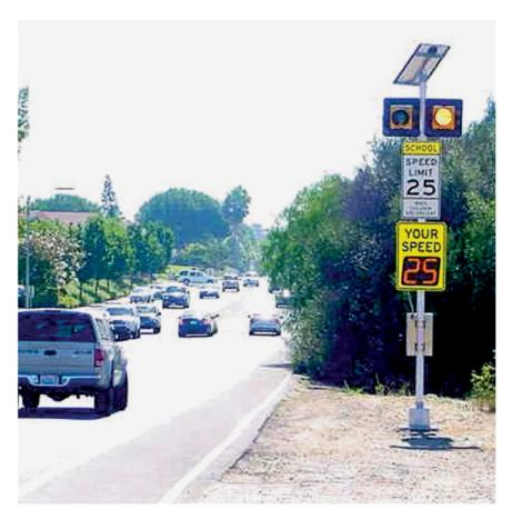
holiday skip periods; and 12 alternate schedule periods. School flashers feature dual 12-inch amber DC flashing beacons to alert motorists to reduced speed limits when flashing. The lamps have an optical output of 1100 candela on center: one of the brightest on the market thus making them more visible in a range of weather conditions especially bright sunlight.
