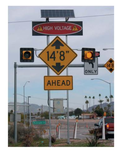
equipment was installed and put into operation at the beginning of March, 2008 and should not require any maintenance on the solar equipment for at least 5 years.
