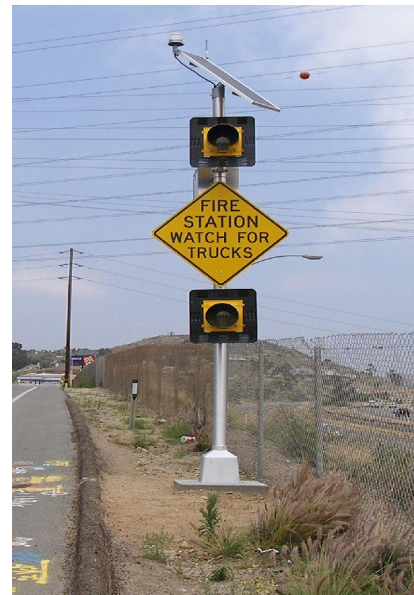
Figure 2 Type I fire station with confirmation strobe beacon
