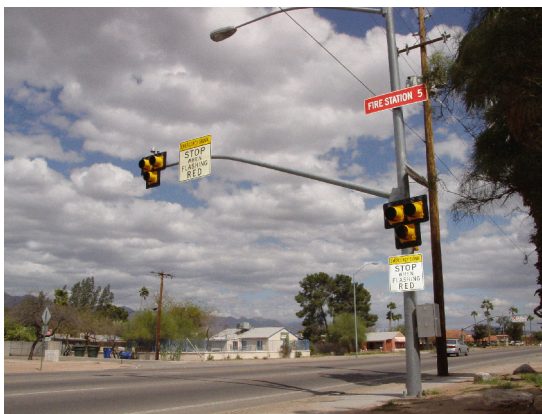
Figure 3 - Type II system installed as a mast arm with type F signal heads
