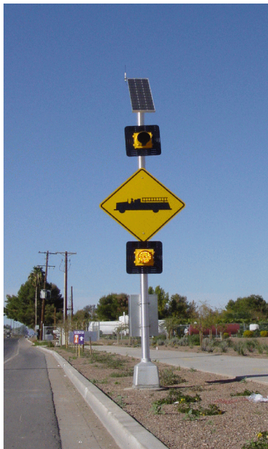
Figure 1 - typical Type I fire station flasher with 2 LED lamps
