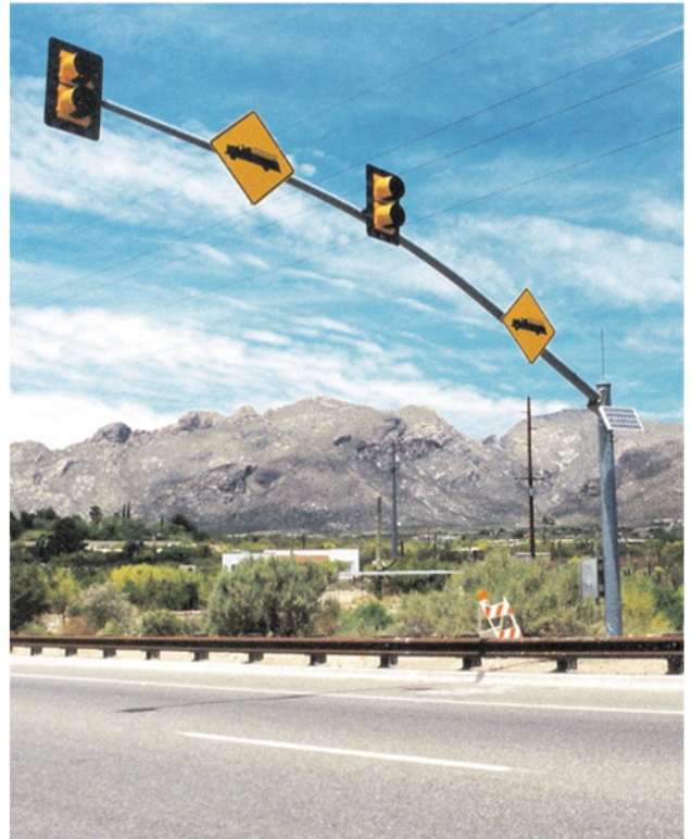
Mast arm installation in advance of fire station with highly-visible warning sign and LED flashers.
